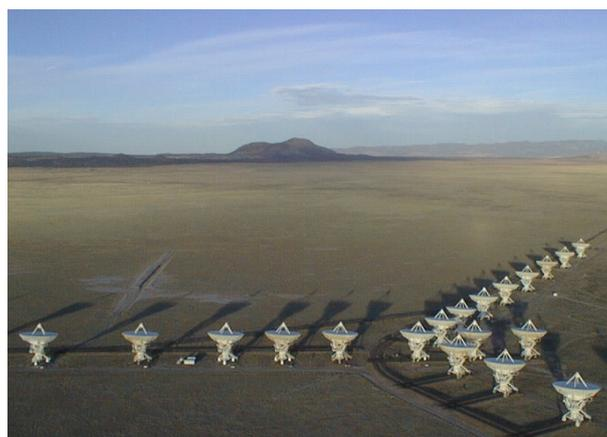
Figure 8.1: The Very Large Array radio telescope in New Mexico. It consists of 27 identical 25-m antennas arranged in a Y-shaped array. Two arms are 21 km long, and the third arm is 19 km long. The array belongs to National Radio Astronomy Observatory, and the picture is taken from <http://www.aoc.nrao.edu>.
